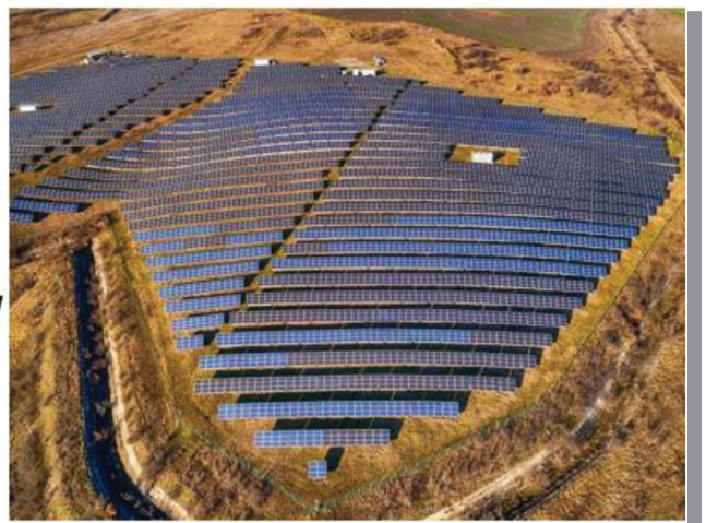
2.8 GW Golmud Solar Park in China ( https://www.theecoexperts.co.uk/solar-panels/biggest-solar-farms )
